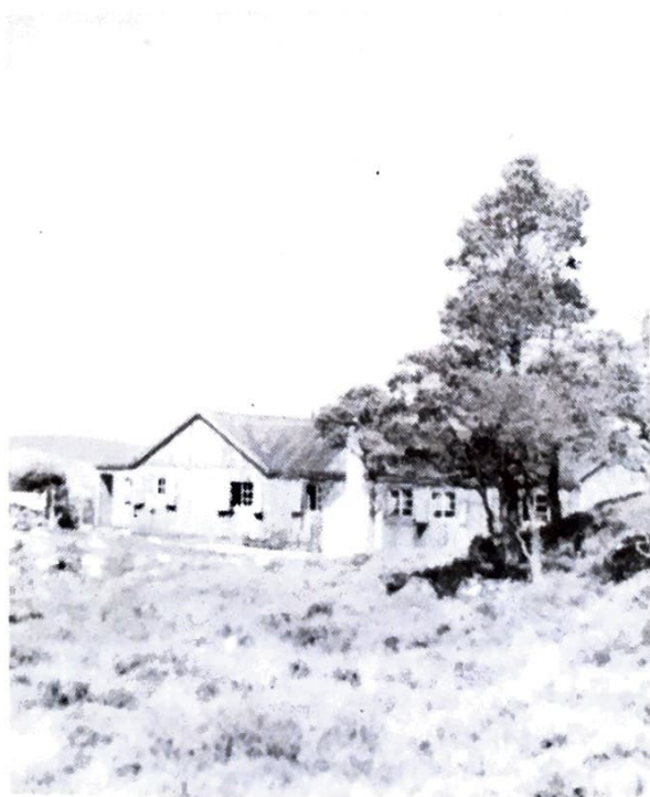
Side view of the original Hut, 1952
